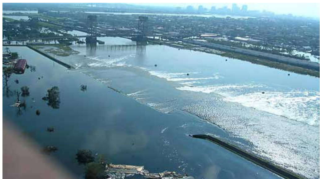
Figure 2. Photo at South Breach of IHNC. (Photo courtesy of USACE.)
