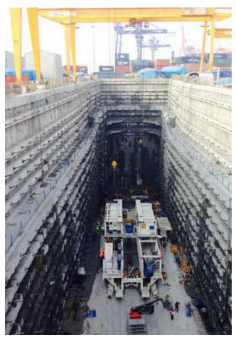
Figure 4. Launch shaft, looking west toward headwall. (Courtesy of Yapı Merkezi, SK E&C JV.)
