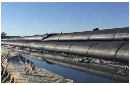
Figure 2. View of geotextile tube wall filled with re-used fly ash in an ash pond at a Mid-Atlantic utility site. (Photo courtesy of TenCate Geosynthetics.)
