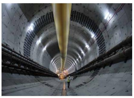
Figure 5. One of the two seismic joints in the tunnel. (Courtesy of Yapı Merkezi, SK E&C JV.)
