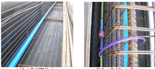
(a) Installed IPI Casing
