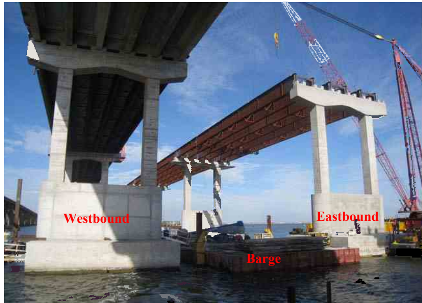
Figure 1. Photo of M19 Eastbound and Westbound Piers Site
